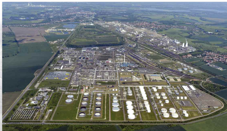
Analytical monitoring of water quality by TOC measurement is essential for efficient processes in the Leuna Chemical
